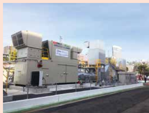
Plant for demonstrating dry low-NOx combustion with a hydrogen-fueled gas turbine
