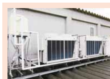
20-HP water-cooled CO 2 condensing unit utilizing waste heat and air-water heat exchanging unit for field tests
