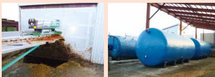
Automatic feeder and pretreatment unit for raw materials as well as an FRP methane fermentation tank (thermophilic dry fermentation)
